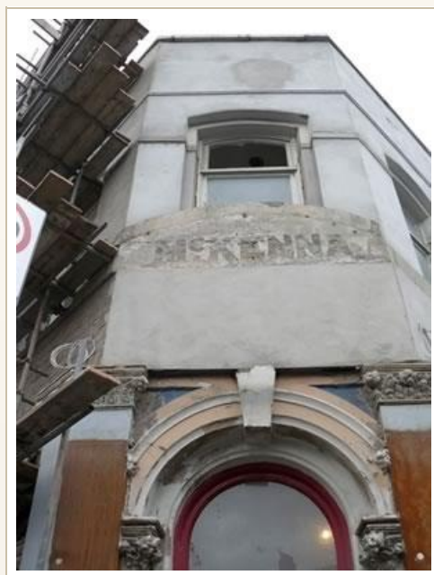
Figure 1 – Evidence of the McKenna ownership above the corner doorway, revealed during
